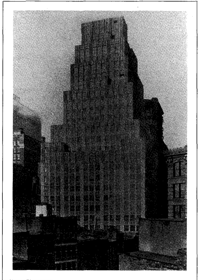
The Insurance Center Building, designed by Ely Jacques Kahn and completed in 1927, illustrates the "wedding cake" architecture that was spawned by New York's height and setback zoning. Source: Avery Architectural and Fine Arts Library, Columbia University in the City of New York.
